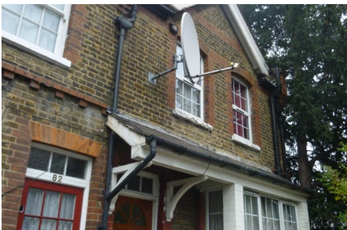
Satellite dish and replacement windows
