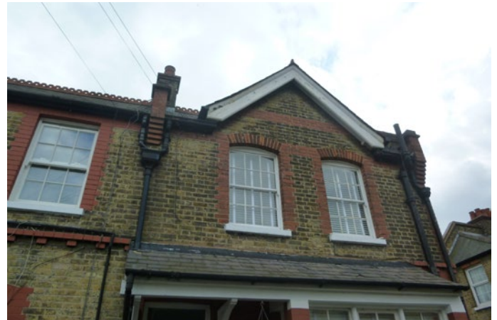
Detail of typical end-of terrace house
